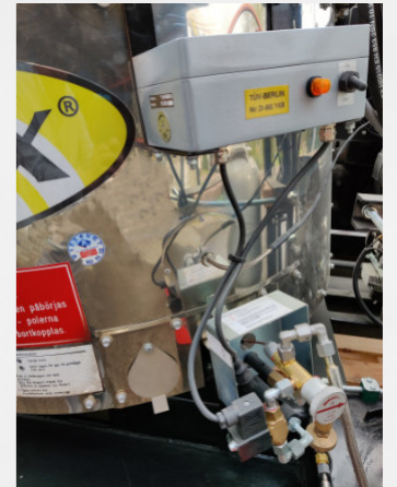
Electronic starting system and FeCuNi temperature sensor
