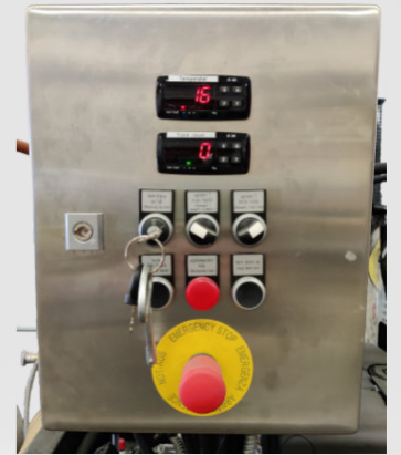
Electronic system control and thermostat
